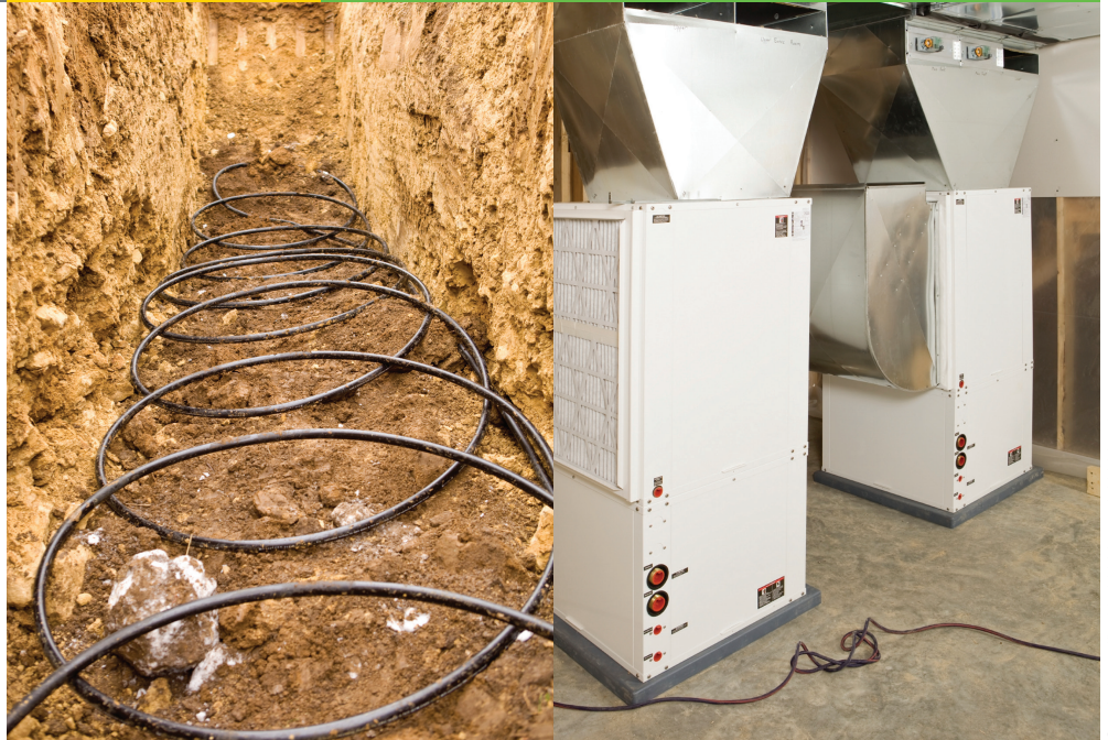
Geothermal heat pump systems, consisting of the heat exchanger (left) and the heat pump (right), heat and cool a home by transferring heat to and from the earth.
